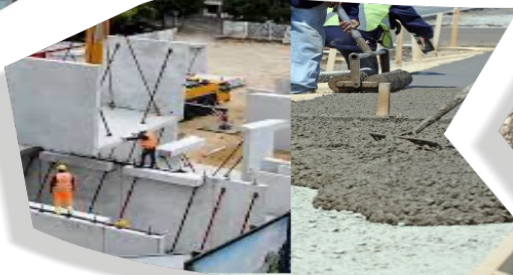
Precast Component/Ready Mix
