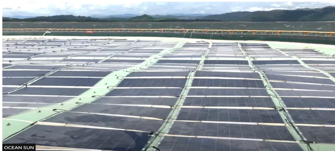
The base of the Ocean Solar plant flexes as waves move underneath it
