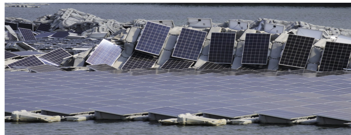
After the outermost row had ripped off the wind-facing edge did not have any ballast anymore to counter uplift from wind. The modules and floaters began to curl-up with the result of an electrical fire.
