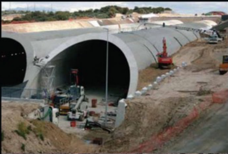
Geotechnical Applications (Retaining Wall, Soil Stability & Foundation)
