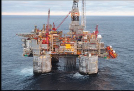
Insulation of Pipeline in Oilfield
