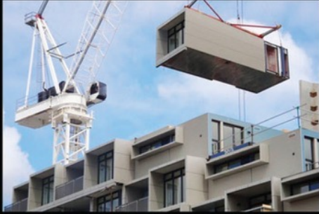
PPVC & PBU Precast
