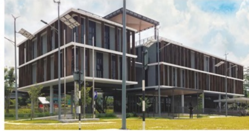
CIDB Complex at Jalan Tampoi, Johor Bahru
