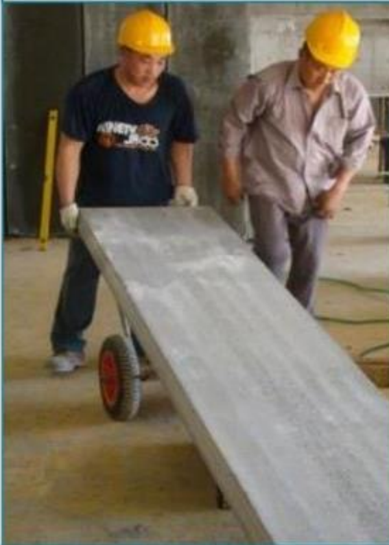
Use Trolley to Move Panel
