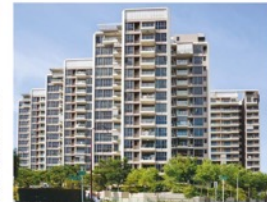
KOVAN REGENCY Condominium
