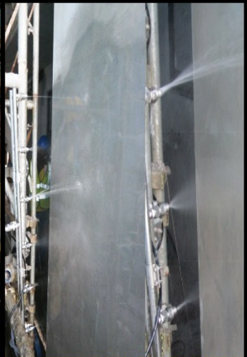
WATER TIGHTNESS TEST Water Seepage = 0%
