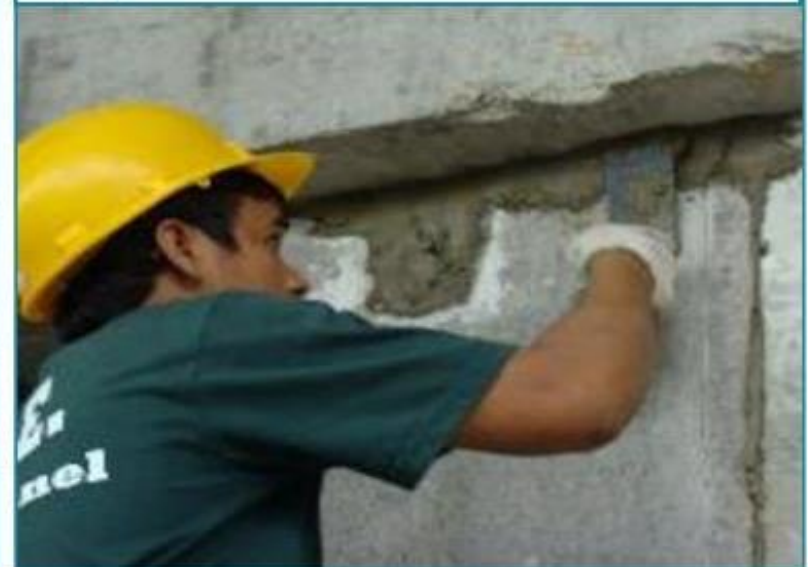
Apply JOE JOINT BONDING Adhesive
