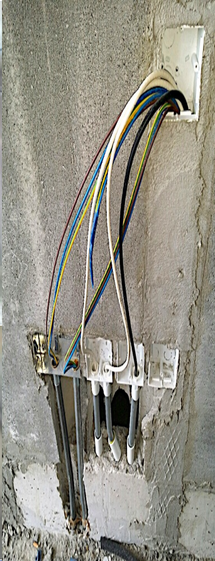
Hollow Core Design for Easy M&E
