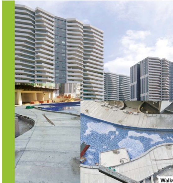
GRANDVIEW 360° Condominium, Johor Bahru, Malaysia
