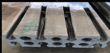
Customized with Rebar & Grout
