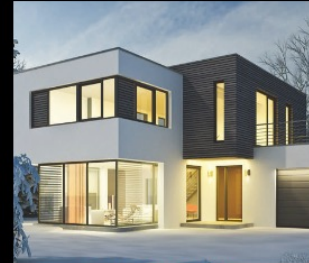
Thermal Insulation (Roofs, Floors, Fire Doors)
