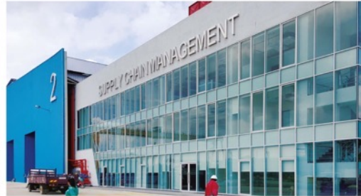
Warehouse, Chemical and Paint Store for Malaysia Marine and Heavy Engineering Sdn Bhd, Johor, Malaysia
