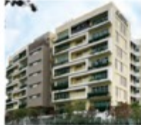
St. Andrew's Nursing Home at Jalan Penjara
