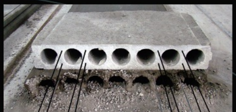
High tensile Wire Reinforcement
