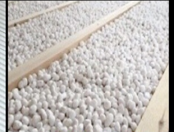
Loose Fill Roof Insulation
