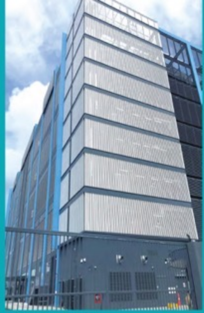
Data Center at Loyang Drive
