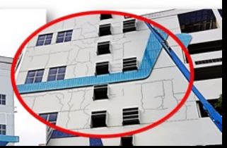
External Cracking
