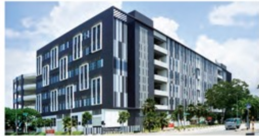
THE WESTCOM at 1 Tuas South Avenue 6
