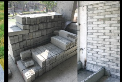
Balance cut to Block
