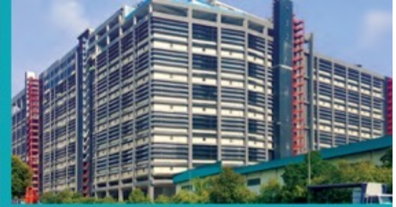
6 Storey Warehouse at 47 Jln Buroh
